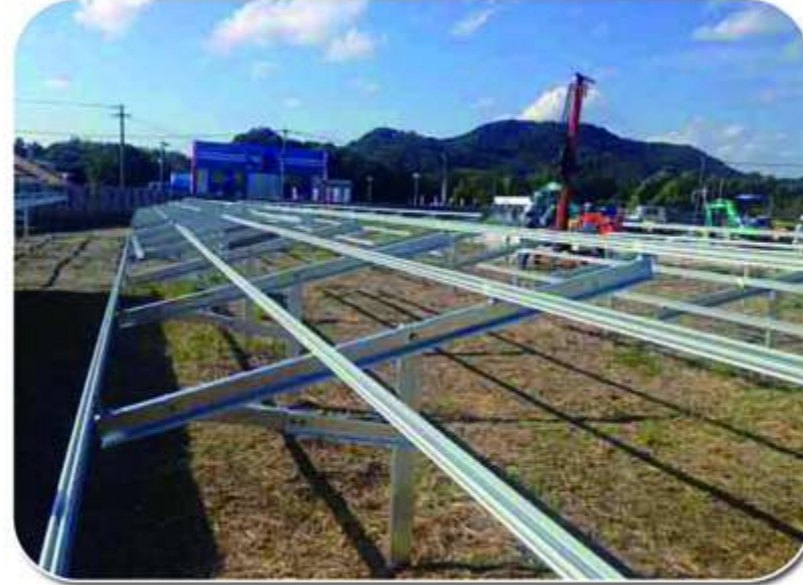
3,5MW SFS-GM-04 Pile Ground Mount Structure(Japan)
